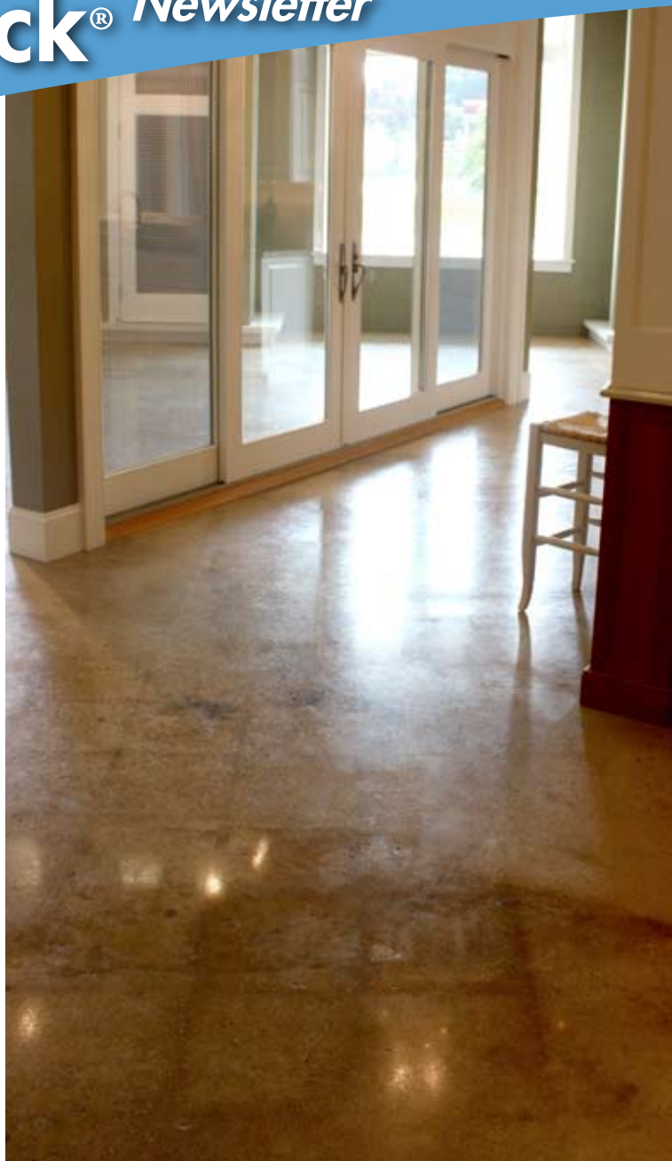
The grid -- Faint and faded, but still there after grinding and multiple polishings and cleanings.
