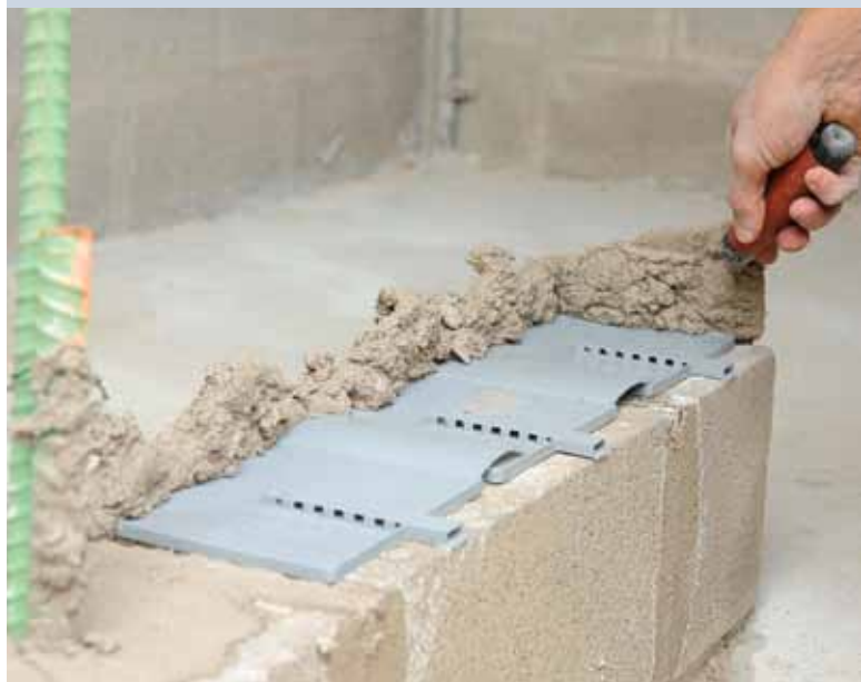
Correcting Kahn’s flashing omission with hidden 2010 technology, one of Cavalieri’s masons grouts the flashing system into place.
